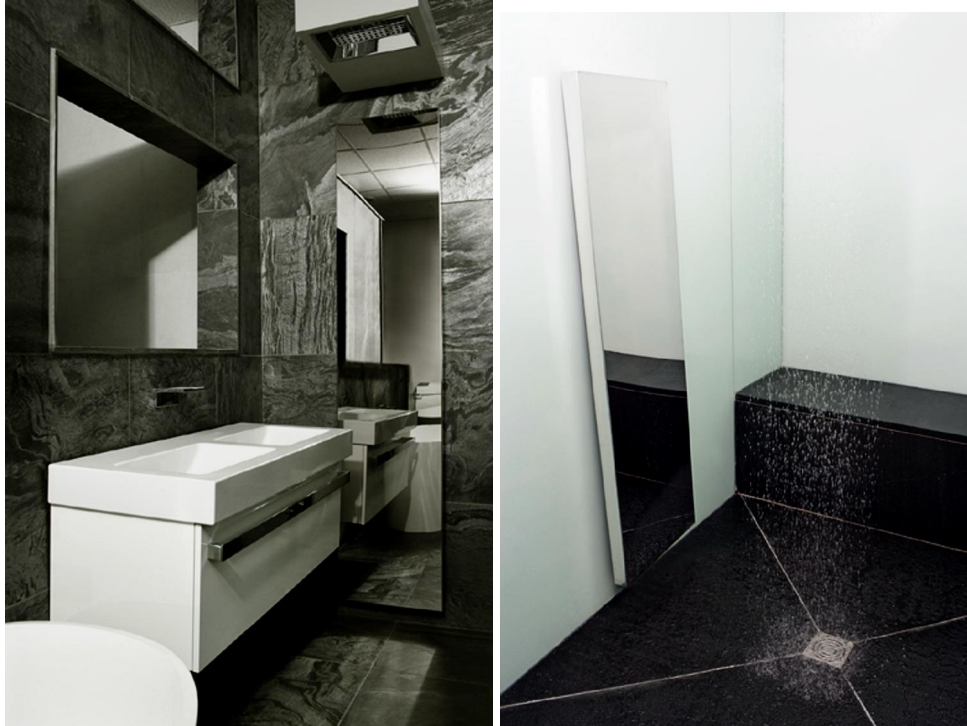
radiators are pictured not plumbed in (without valves)
